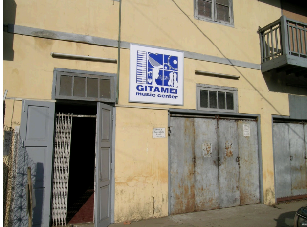
Figure 1 Building of Birth: 2003, Taumwe township Yangon
